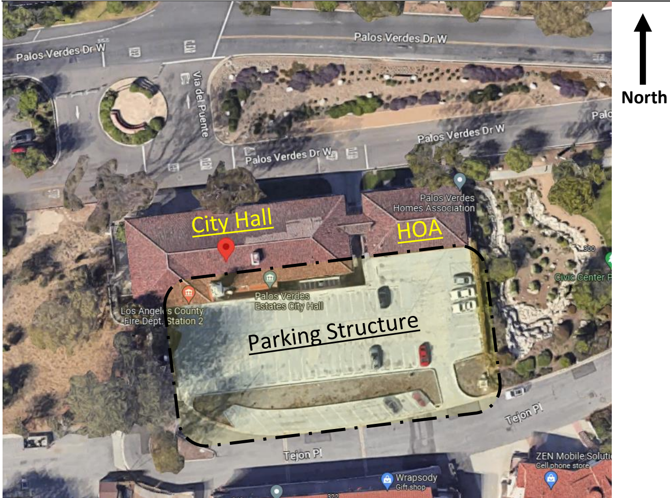
Figure 1 - Aerial view of the City Hall Buildings (Google Maps)
