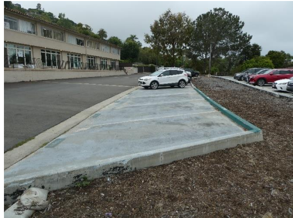
Photo 8 - Condition of the surface parking adjacent to the □□□
