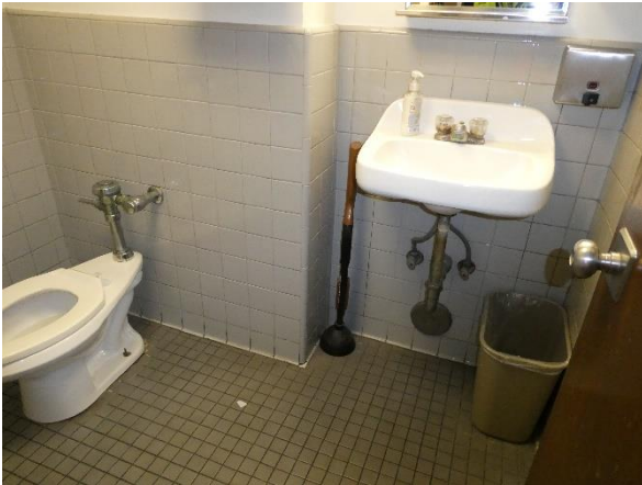
Photo 115 - Building 340 (Police Department): Bathroom.
