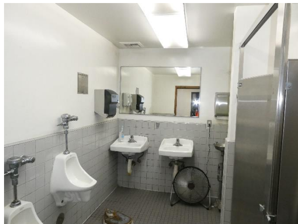
Photo 108 - Garage restroom finishes.
