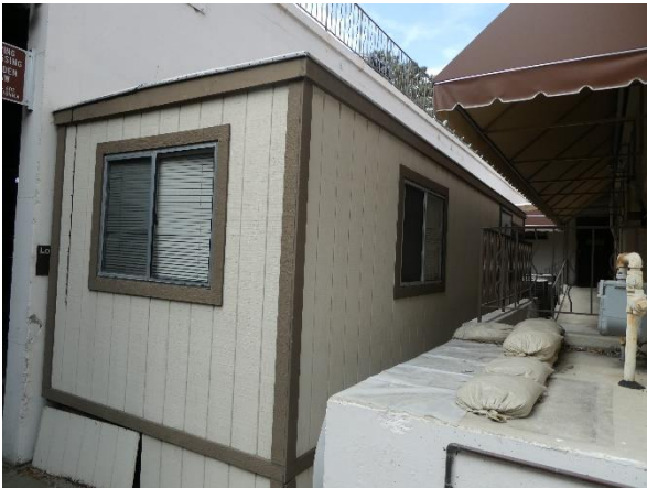
Photo 111 - Freestanding building adjacent to Building 340.
