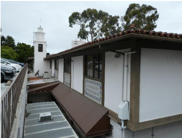
Photo 51 - Building 340: South elevation.
