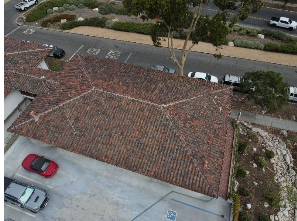
Photo 70 - Building 320: Roof overview.
