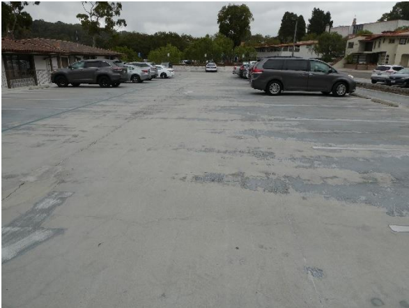
Photo 7 - Overview of the condition of the parking □
