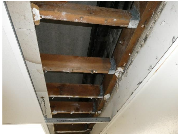
Photo 100 - Building 320 (Maintenance Department): Upper-level floor system as viewed from below.
