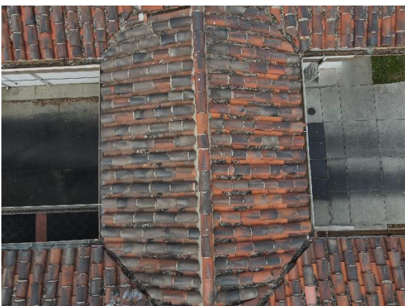
Photo 77 - Overview of walkway roof.
