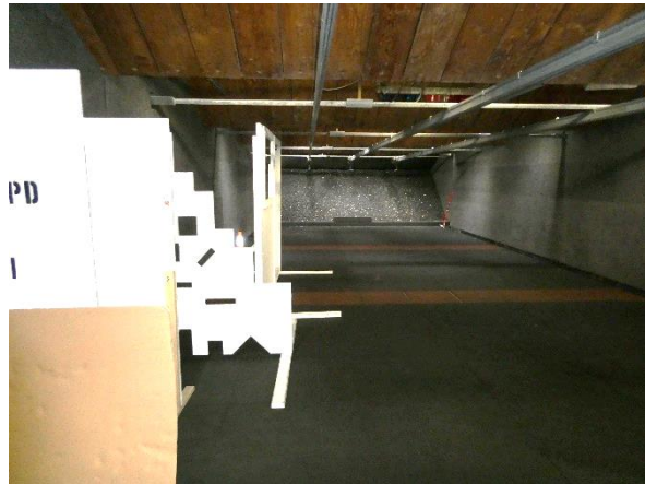
Photo 118 - Building 340 (Police Department): Shooting range.
