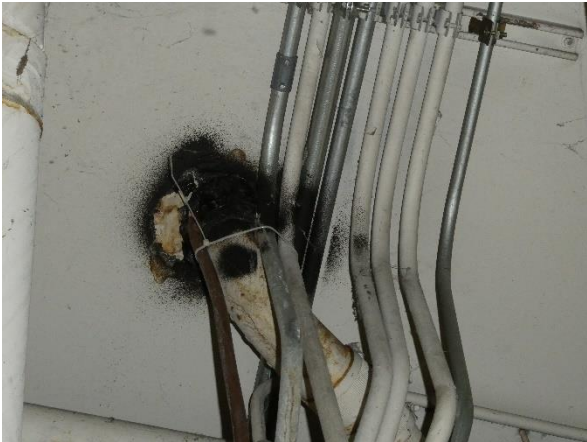
Photo 109 - Garage: Repair to drain.
