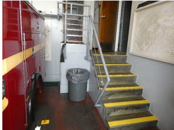
Photo 122 - Building 340 (Fire Station): Stairs leading to office and living area.
