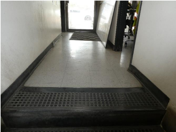
Photo 97 - Building 320 (Maintenance Department): Corridor finishes.
