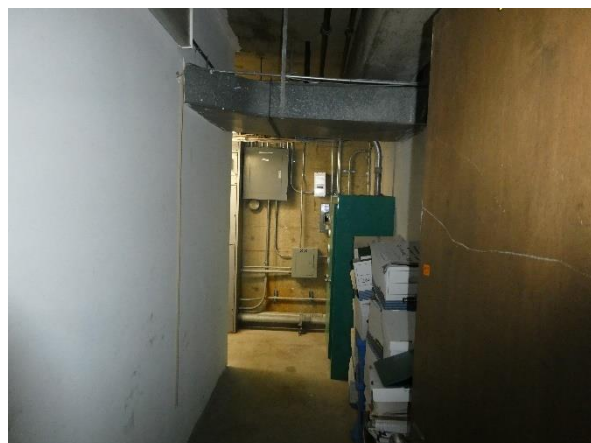
Photo 102 - Building 320: Basement corridor finishes.
