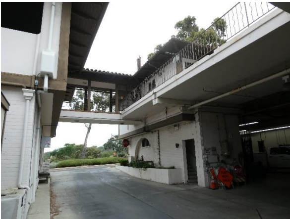
Photo 29 - Building 320: West elevation.
