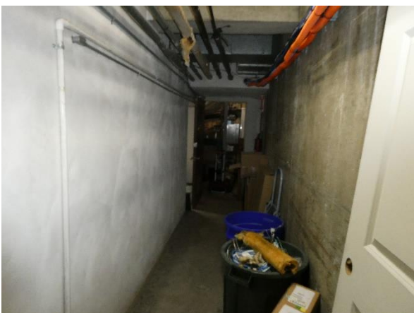
Photo 101 - Building 320: Basement corridor finishes.
