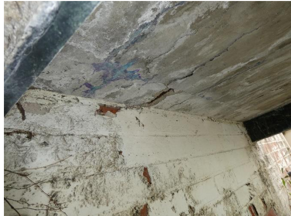
Photo 28 - Condition of cast-in-place concrete at the water feature.
