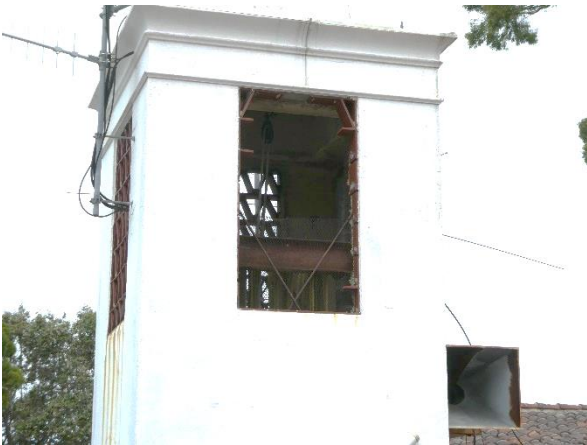
Photo 57 - Building 340: Missing tiles at the tower.
