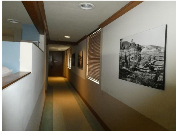
Photo 128 - Building 340 (City Hall): Corridor finishes.
