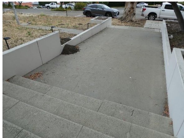
Photo 166 - An accessible path from the municipal sidewalks to City Hall entrance from Palos Verdes Drive West is not provided.
