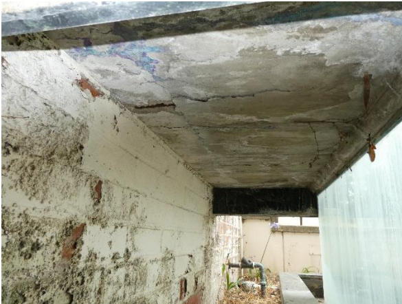
Photo 27 - Condition of cast-in-place concrete at the water feature.
