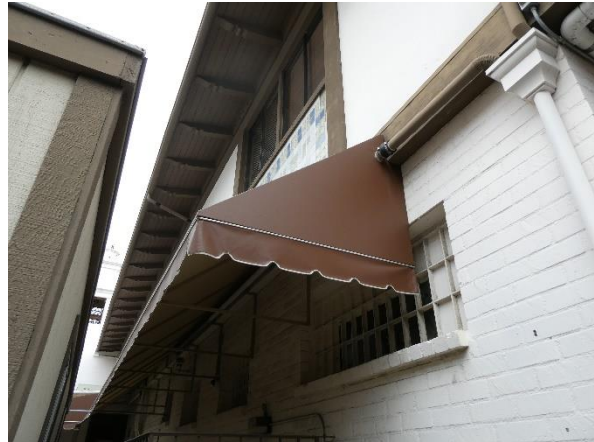
Photo 50 - Building 340: Vinyl-wrapped, metal-framed awning at the South building elevation.
