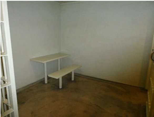
Photo 117 - Building 340 (Police Department): Holding cell.
