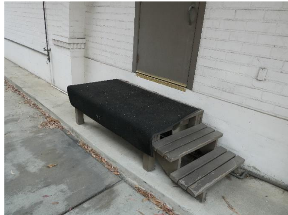
Photo 52 - Building 340: The stair assembly at the east elevation employee entrance.
