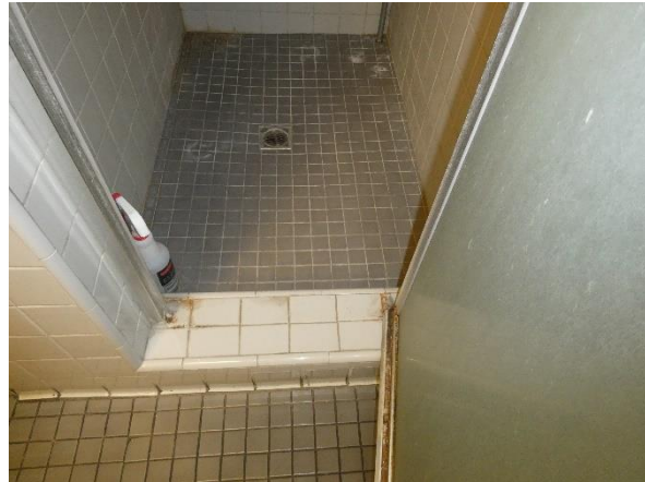
Photo 116 - Building 340 (Police Department): Shower finishes at bathroom.
