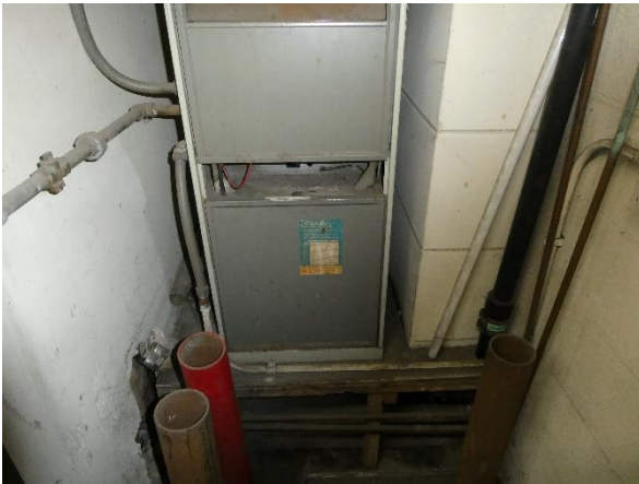
Photo 135 - Building 320: Original furnace in the basement.
