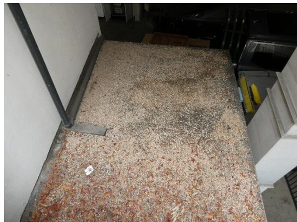
Photo 90 - Building 340: Condition of the built-up roof at the garage.
