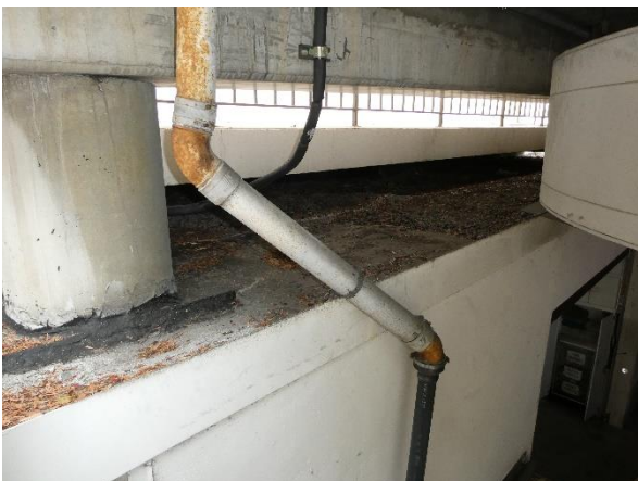
Photo 89 - Building 340: Condition of the built-up roof at the garage.
