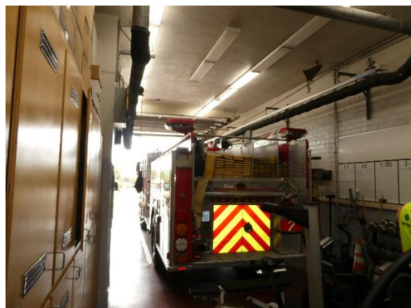
Photo 120 - Building 340 (Fire Station): Interior finishes.
