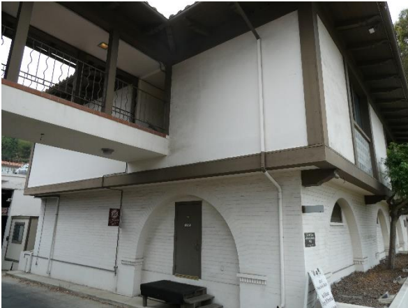
Photo 49 - Building 340: East elevation.
