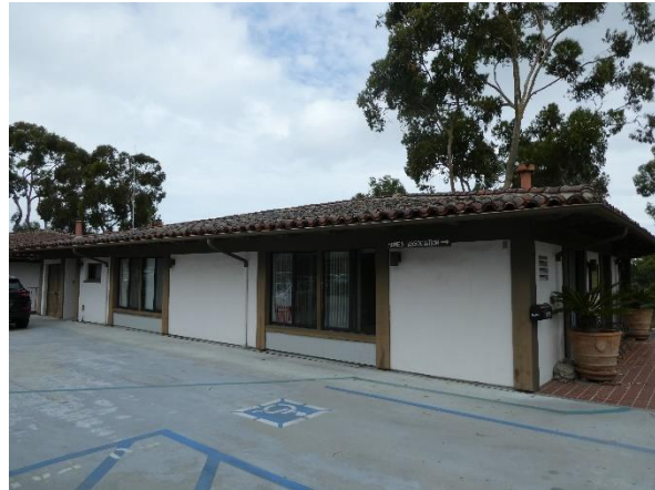
Photo 32 - Building 320: South elevation.
