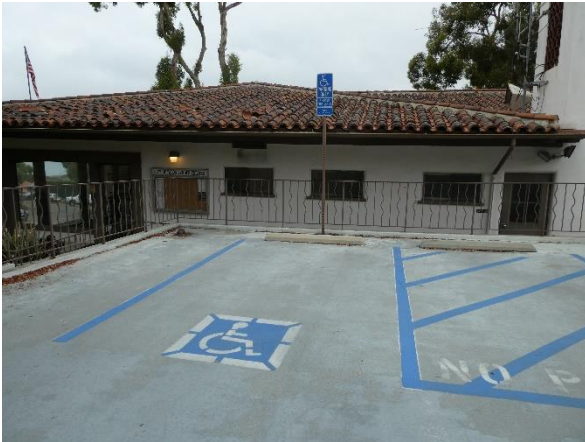
Photo 163 - Building 340: Accessible parking space.
