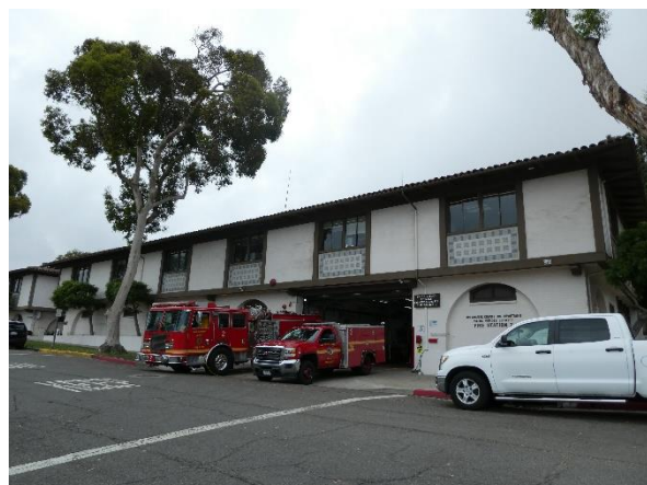
Photo 48 - Building 340: North elevation.
