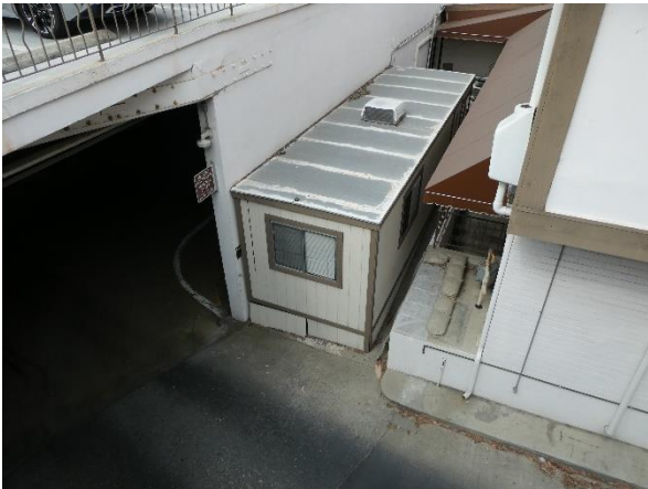
Photo 75 - Freestanding building adjacent to Building 340
