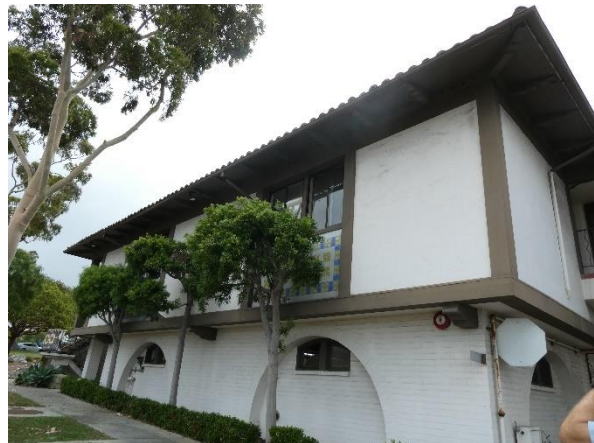
Photo 30 - Building 320: North elevation.
